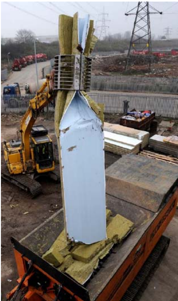
Figure 3: Composite panel being fed into a composite panel recycling machine (Eurobond)
